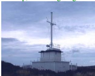
Rooftop mounted 'Naval' mast.
