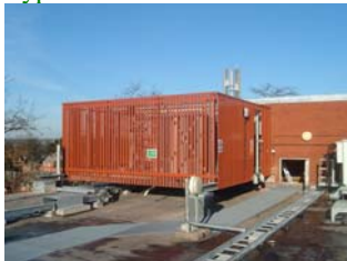
Rooftop, screened grillage
